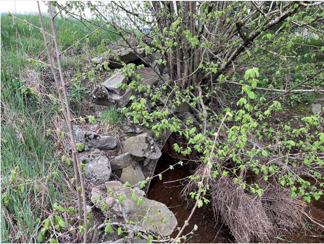
Culvert Outlet (South End)
