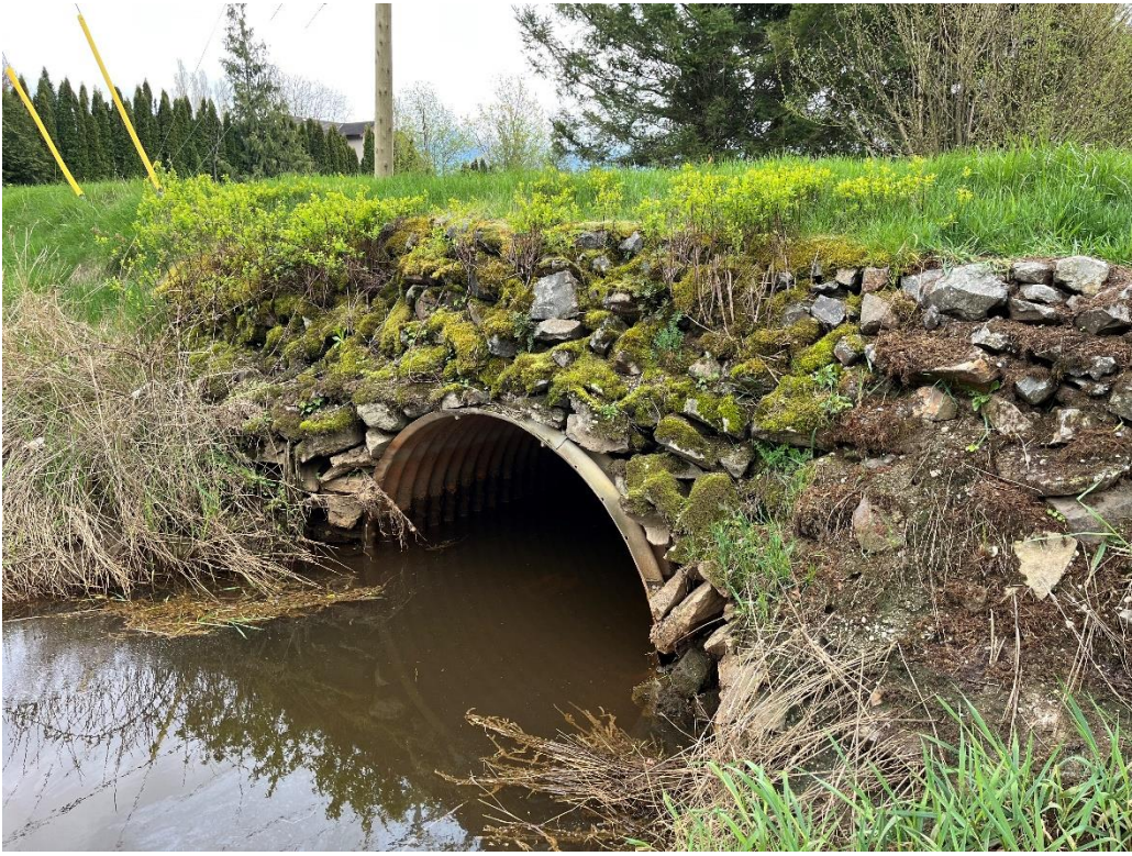
Culvert Inlet (North End)
