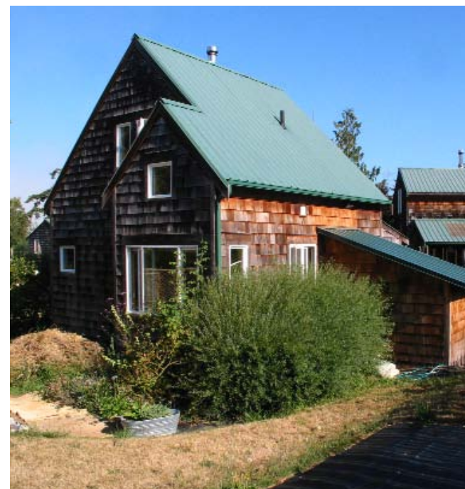
Newer construction can reflect the lines of historic homes and maintain a sense of the islands' past.
