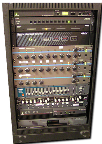
The Council Chambers switching rack holds all A/V filtering and switching equipment.
