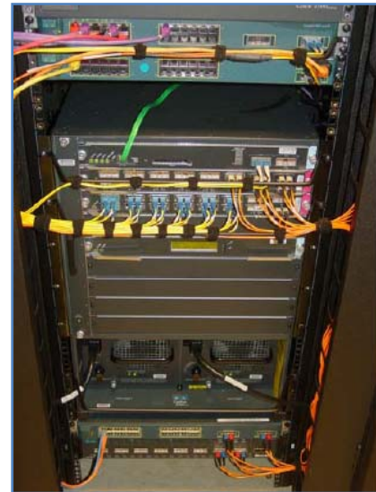
Central Switch at School District Data Center
